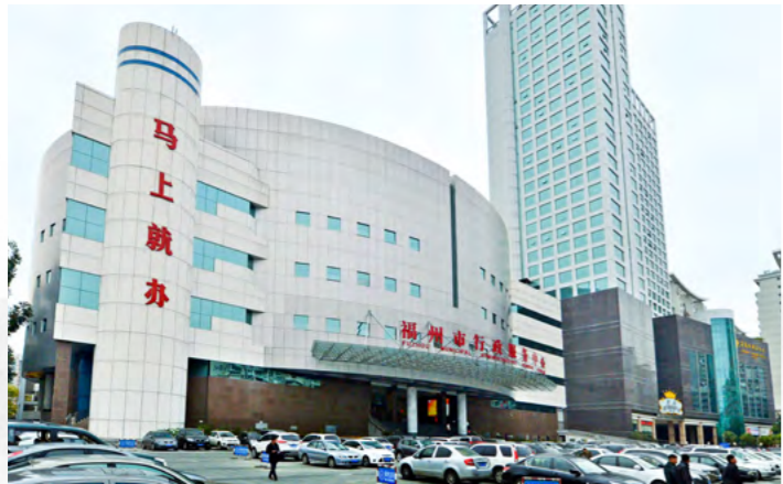
Administrative service center of Fuzhou
