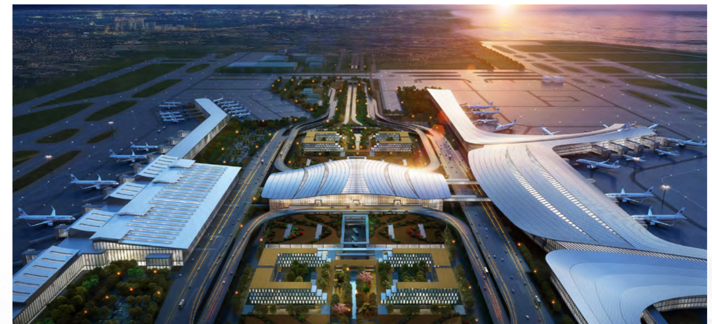
● Changle International Airport: the international airport with the best clearance conditions nationwide
