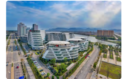
● Southeast Big Data Industrial Park
