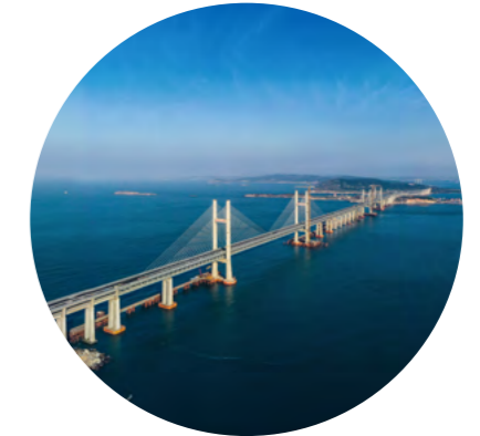
Pingtan Strait Highway-Railway Bridge
